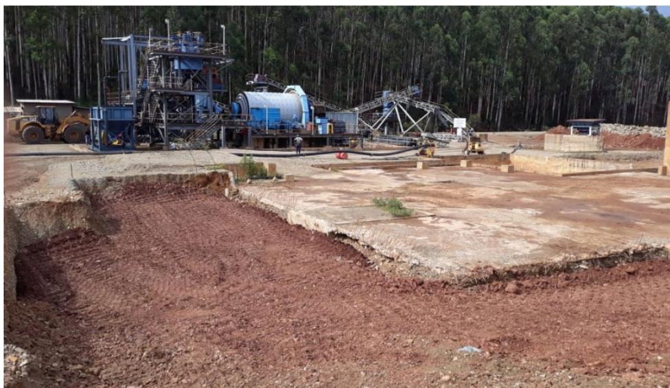
**Image 2.** First Fill and Compaction in CIL Area
